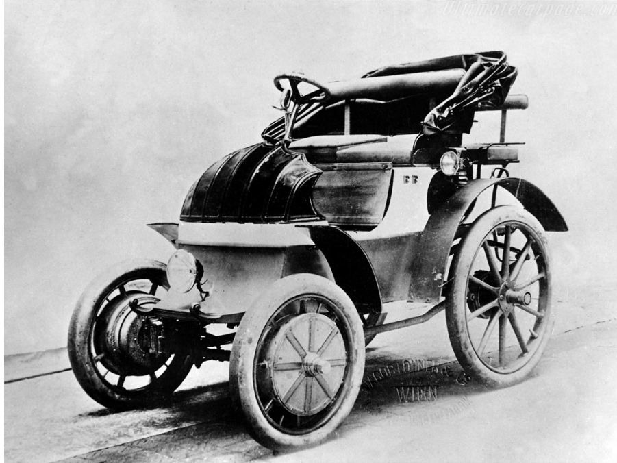
Figure 2: An early 1900s 'System Lohner-Porsche', propelled by in-wheel motors [34]
